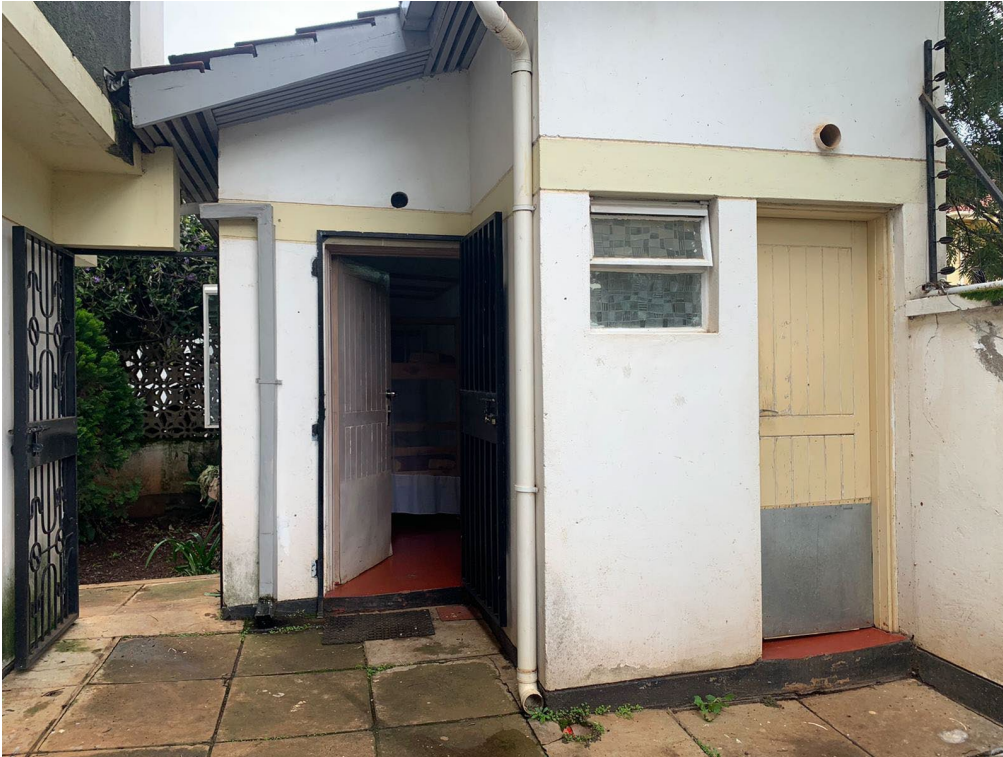
SQ room exterior & bathroom exterior
